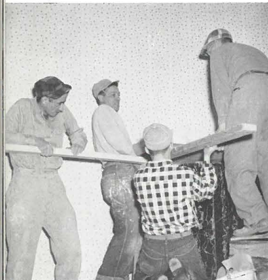
MARBLE-SETTERS hold their breath as they lower the two-ton altar top into place.
